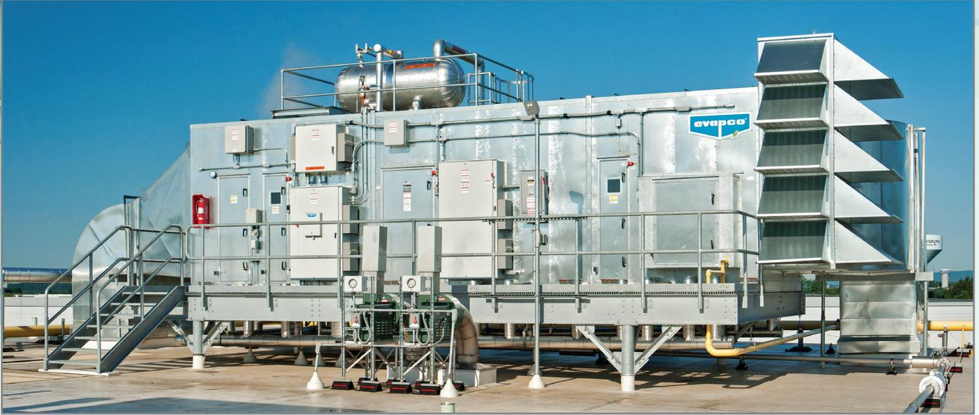
Critical Process Air (CPA) Hygienic Air Handling System
