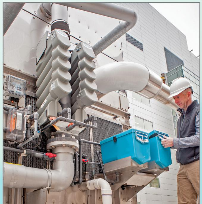
Smart Shield® Factory-Mounted Water Treatment System
